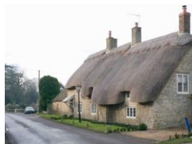
Example of building frontage set directly against public grass verge
