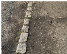
Kerb to footway of granite setts
